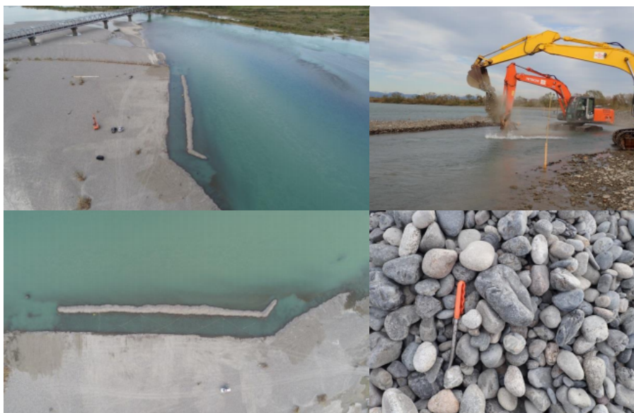
Fig. 9. Diagonal and vertical aerial shots taken immediately after the completion of construction on November 1, 2018 (top and lower left); Throwing of gravel and gravel thrown in the channel (top and lower right).
