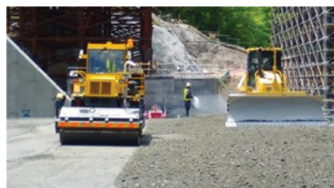
Figure 4. Bulldozer and vibrating roller with GNSS
