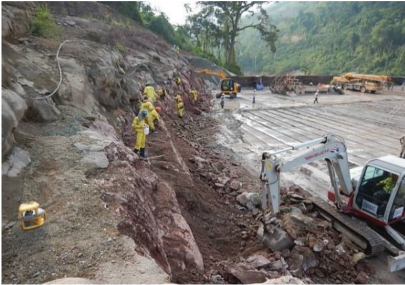
Figure 8. Rock foundation excavation and treatment
