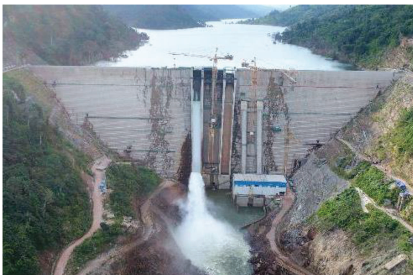
Figure 1. RCC dam in NNP1 in November 2018
