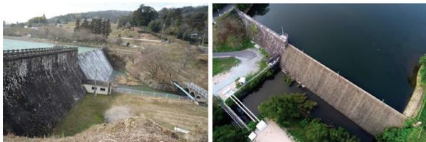
Figure 10. Photograph views of Senbon Dam: the sharp edge of the dam top creates hydraulic beauty.
