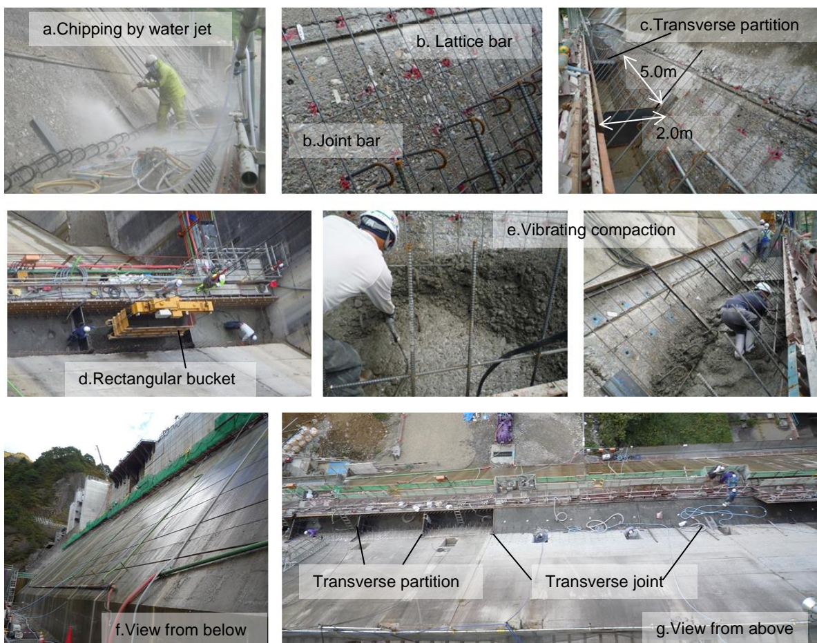
Figure 7. Situation of concrete placing on the downstream surface
