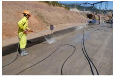
2. Green-cut using high pressure jetting
