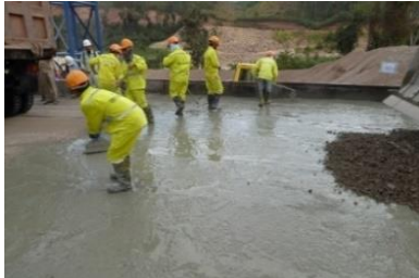
4. Bedding grout (3 mm thick)
