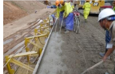
6. GE-RCC compaction
