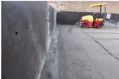
7. Compaction of RCC by large roller (RCC and GE-RCC at interface)
