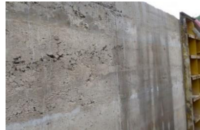
9. After removal of formwork(left no GE-RCC and right GE-RCC)
