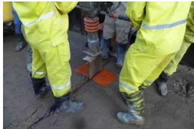
8. Creating contraction joint
