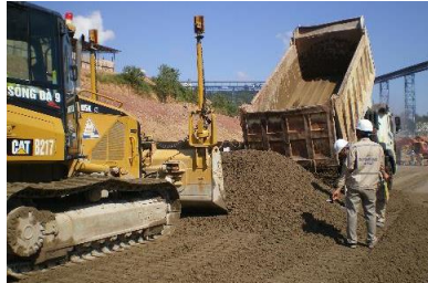
5. Dumping RCC and levelling
