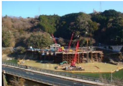
Figure 1. Underwater construction using the fence to prevent turbid water diffusion
