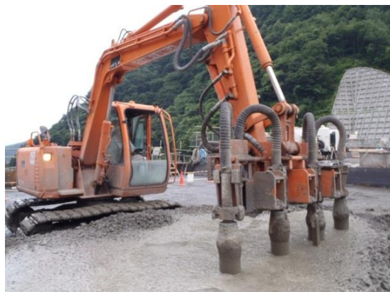
Figure 1. Compaction of dam concrete (using Viback with four vibrators)
