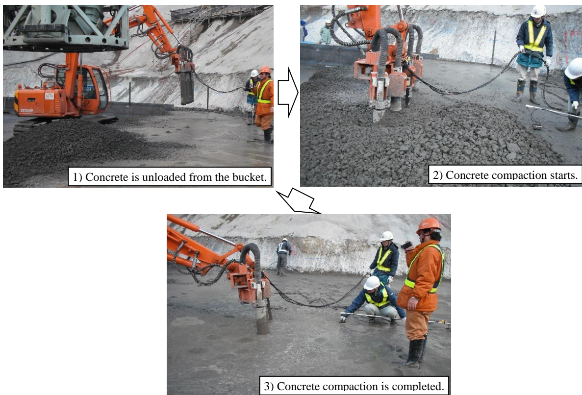
Figure 2. The compaction situation of the dam concrete
