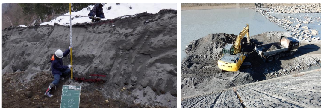
Figure 10. Removal of volcanic products deposited in the sediment trap dam (February 4, 2015)
