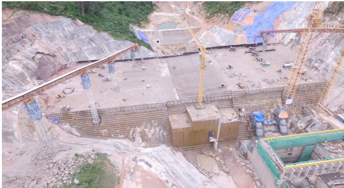
Figure 13 State of Concrete Placing at Dam (December 2016)
