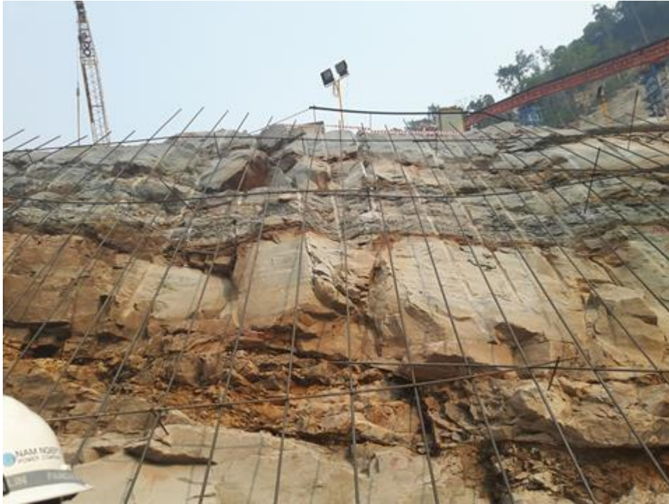
Figure 12. Photo of Re-Bar Installation
