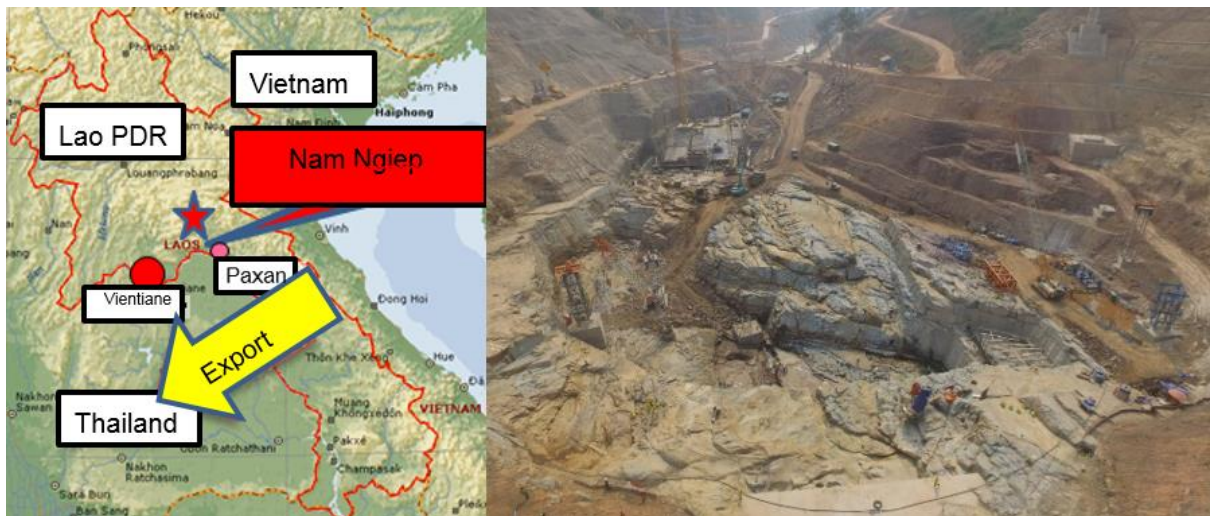
Figure 1. Location Map of Nam Ngiep 1 and Current Status of Excavation
