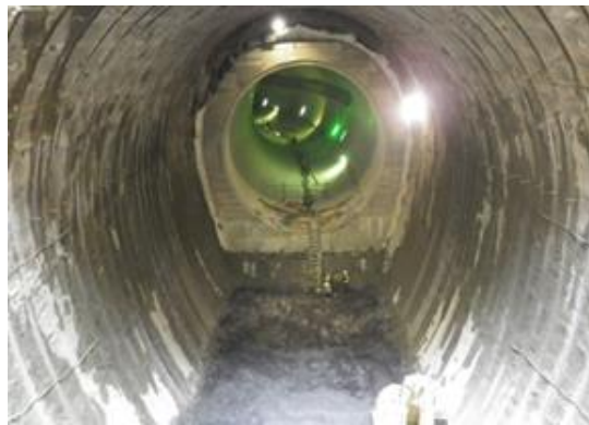
Figure 17. Completion of excavation at the bottom slab
