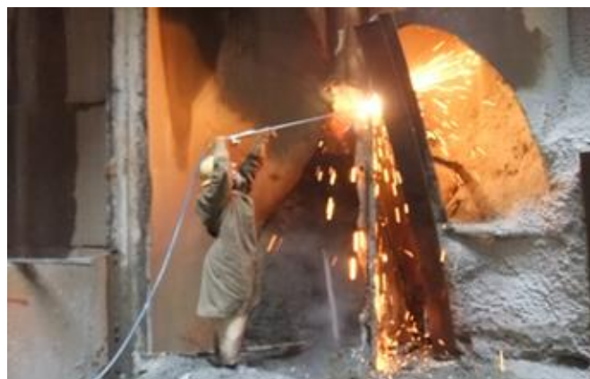
Figure 16. Cutting with the oxygen lance
