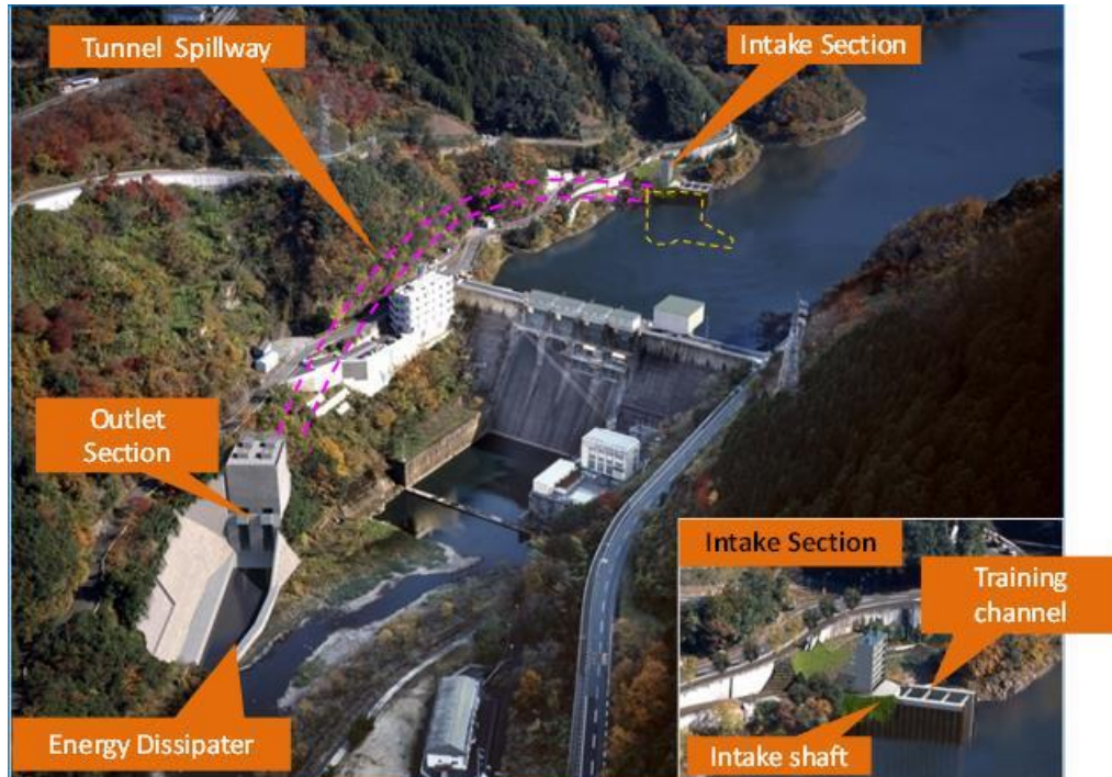
Figure 3. Overview of tunnel spillway
