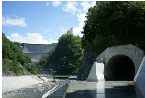
Figure 6. Outlet of the Koshiu dam SBT
