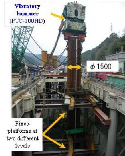
Figure 11. Erection of steel pipe sheet piles using a vibratory hammer
