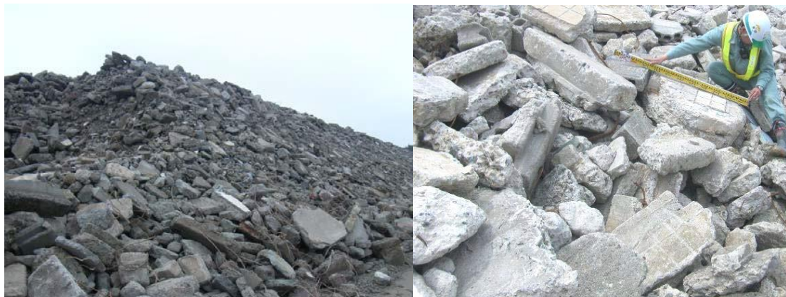
Figure 11. Condition of concrete gravel base material
