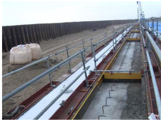
Figure 14. Construction of protection concrete joint
