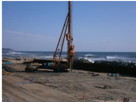
Figure 16. Construction of sand compaction pile
