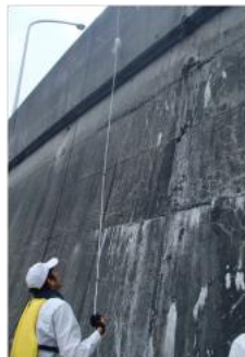
Figure 17. Installing a marker rope
