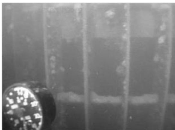
Figure 12. Screen for the stand-by gate of the outlet works of the Yagisawa Dam
