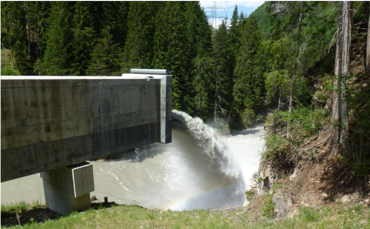
Figure 8. Outlet of the Solis SBT (courtesy of C Auel).
