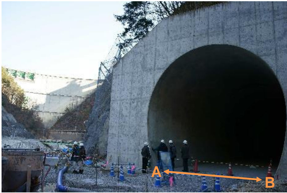
Figure 11. Outlet of the Koshibu dam SBT
