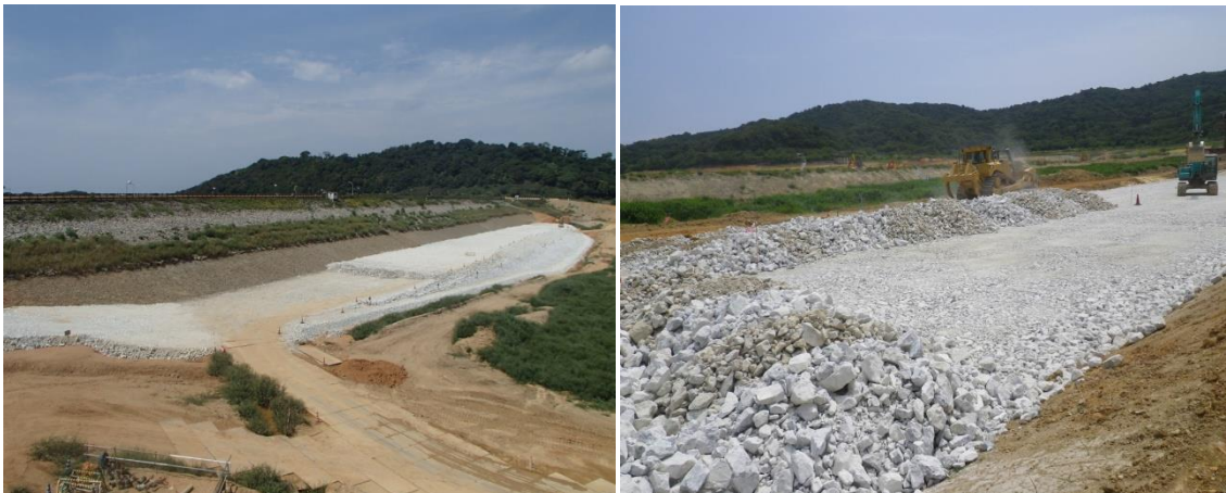
Figure 17. The upstream side of the embankment
