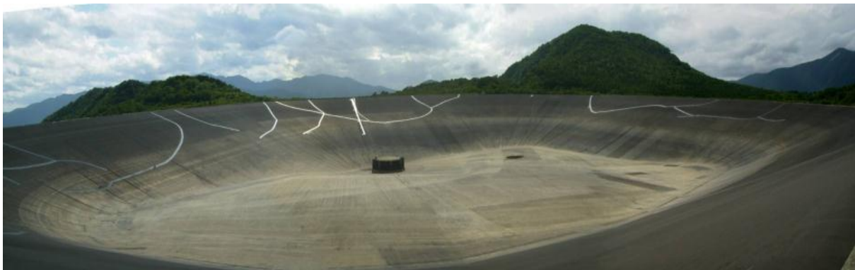
Figure 11. Panorama View of Repair Works Completion (2011.6)
