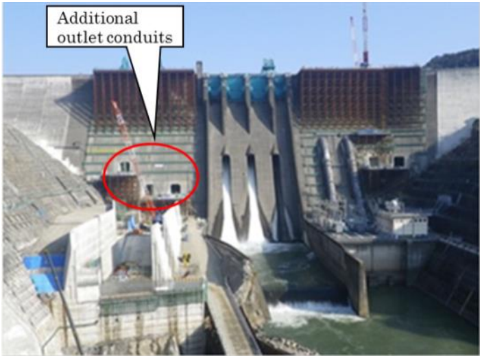
Figure 6. Tsuruda Dam Redevelopment Work (now in progress)
