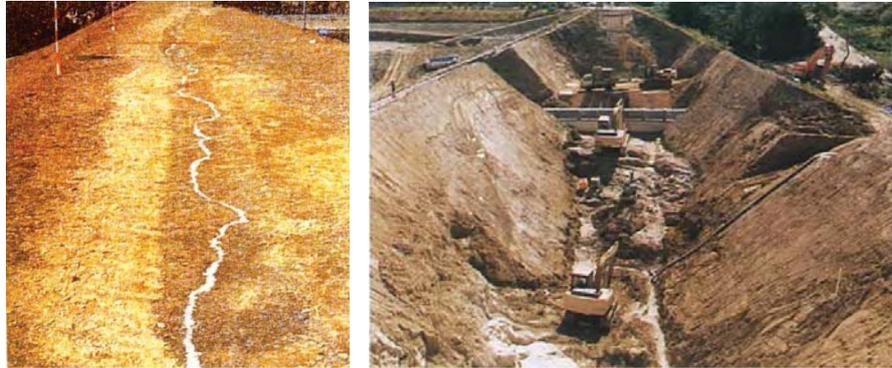
**Figure 2.** Crack on the crest (left) and repairing work (right) of the Kinjoike dam after the Kobe earthquake in 1995 (Hyogo Prefecture, 1996)
