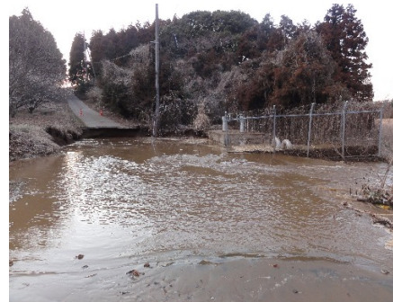
Photo 2. Water leakage from pipeline systems
