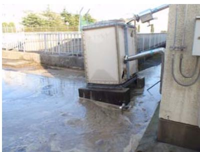
Photo 3. Subsidence caused by liquefaction
