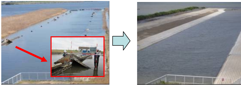
Photo 8. Disaster recovery (left) damaged bank protection (right) after recovery
