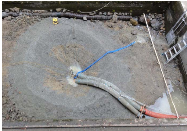
After sediment discharge
