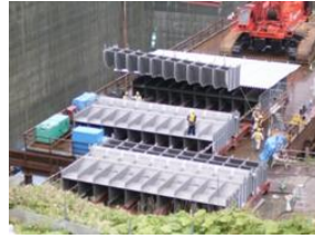
Figure 20. Intake Pipe In-situ Assembly
