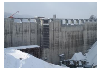
Figure 25. Yubari Shuparo Dam Intake Facilities
