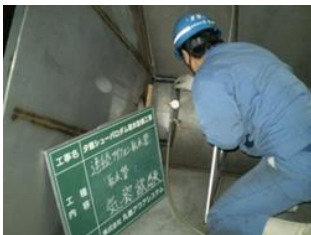
Figure 13. Intake Pipe Airtightness Test
