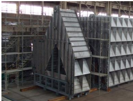
Figure 16. Bottom Intake Pipe Temporary Assembly
