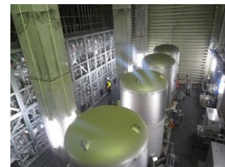
Figure 24. Receiver Tank Installation
