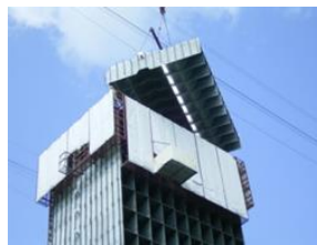
Figure 21. Intake Pipe Lowering In
