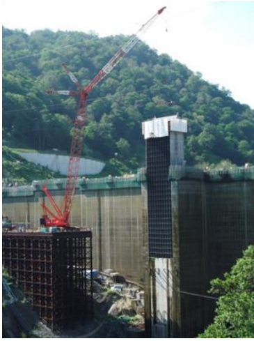
Figure 19. Intake Pipe Installation
