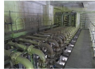
Figure 23. Air Pipe Installation
