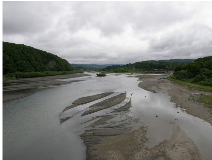
Figure 1. Accumulated Sediment in Nibutani Dam
