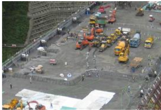
Photo 4. Stopping placing with 1:08 end-slope in cruising RCD construction method
