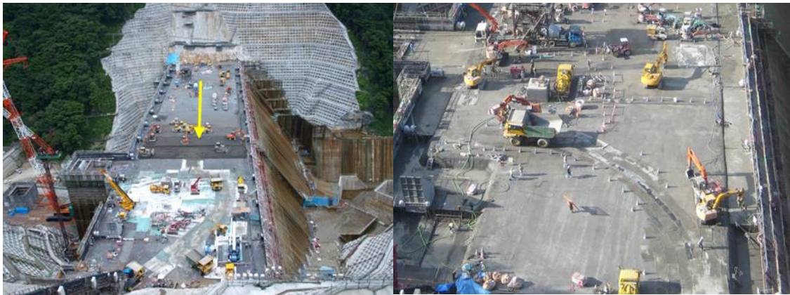
Photo 1. View of cruising RCD construction method
