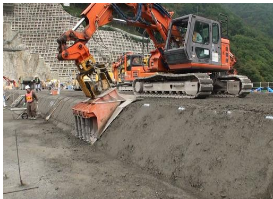
Photo 3. Compacting end slope of RCD concrete
