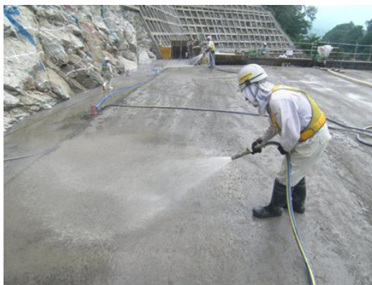
Photo 5. Soft treatment for RCD concrete placing joint surface
