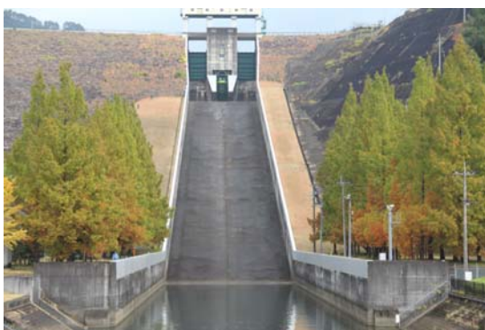
(a) Spillway Seen from Downstream
