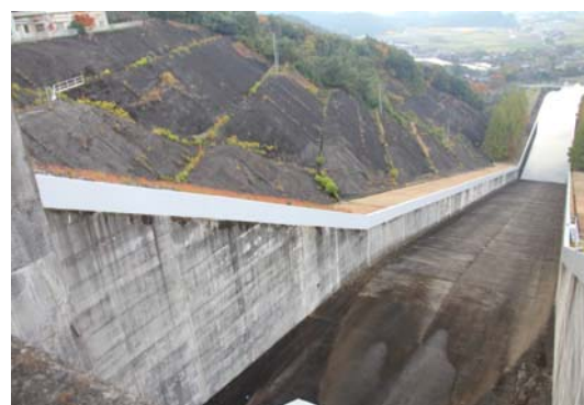
(b) Spillway Seen from Upstream
