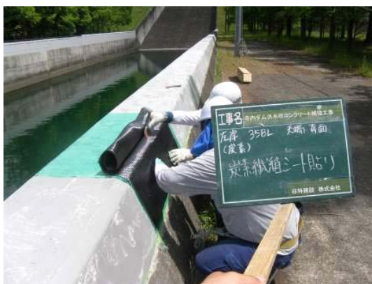
(b) Carbon Fiber Sheet-Affixing Work
