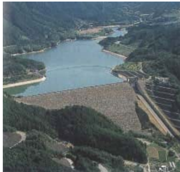
Figure 2. Panoramic View of Terauchi Dam.
