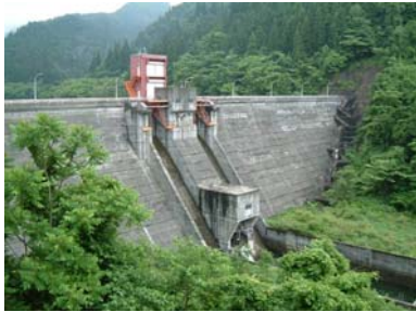
Figure 4. Downstream View of the Tobe Dam (Before Reconstruction).
