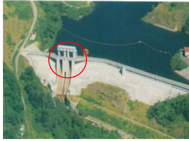
Figure 7. Panoramic View of the Bibai Dam (Before Reconstruction).
