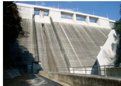
Figure 2. Downstream View of the Sugo Dam (After Reconstruction)
