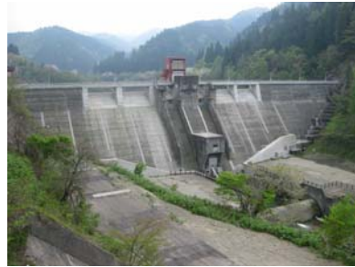
Figure 5. Downstream View of the Tobe Dam (After Reconstruction).
