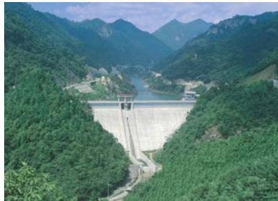
Figure 1. Panoramic View of the Sugo Dam (Before Reconstruction)
