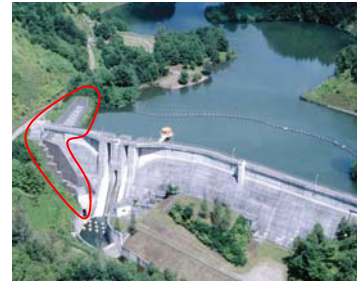
Figure 8. Panoramic View of the Bibai Dam (After Reconstruction).
