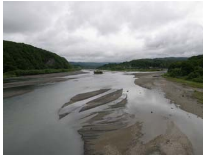
Figure 1. Accumulated Sediment in Nibutani Dam.
