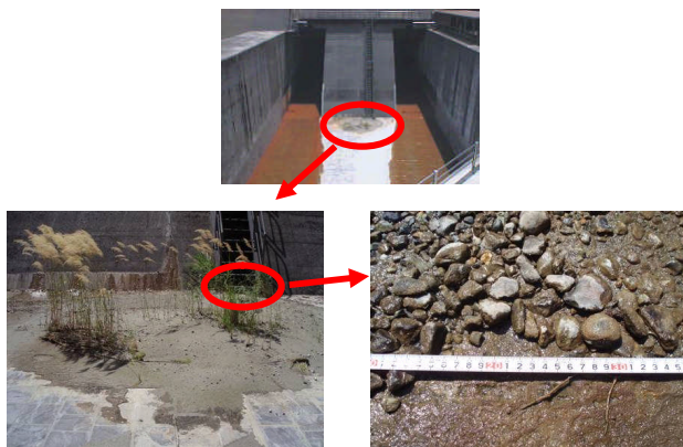
Figure 10. Remained Sediment at the Lower End of the Gate
