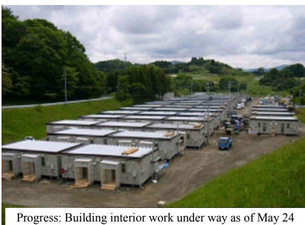
Figure 10. Land for temporary housing near Miharu Dam
