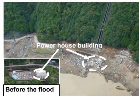
Figure 4. Collapsed Nagatono power plant
