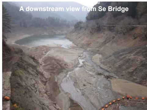
Figure 13. Sedimentation in Asahi Dam
