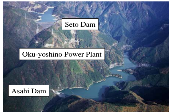
Figure 7. A view of the Okuyoshino Power Plant
