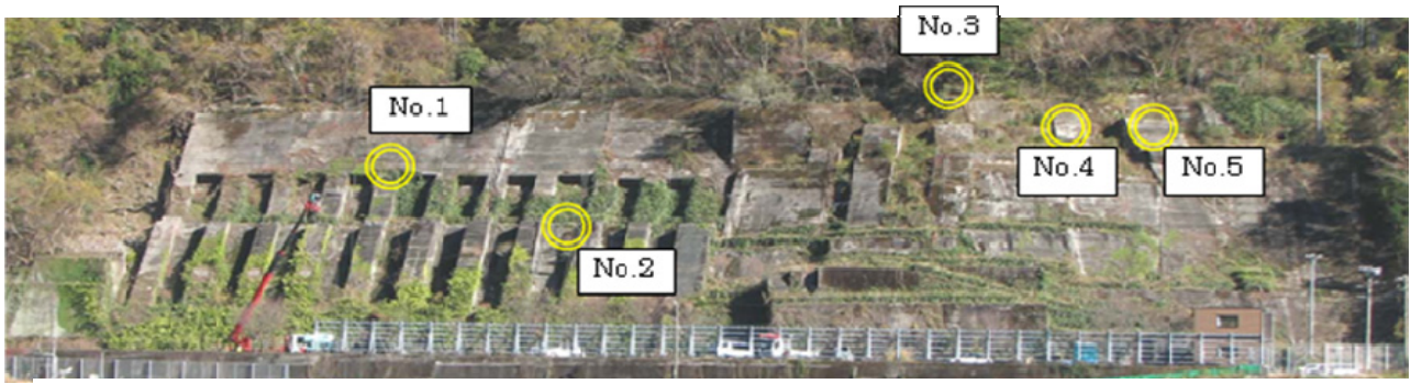
Figure 6. Retaining wall (double circle indicates locations of crack extensometers)
