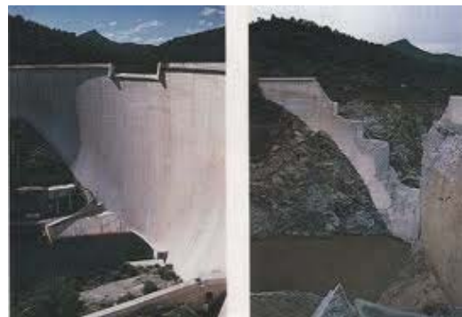
Figure 1. Malpasset dam (before and after the collapse, MA 1960)
