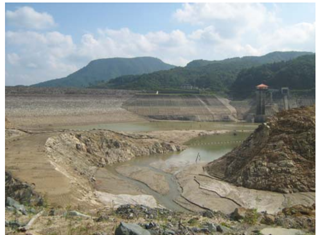
Figure 12. Upstream view of the right side of the Aratozawa dam and reservoir bottom when the reservoir water level was lowered in September, 2008.
