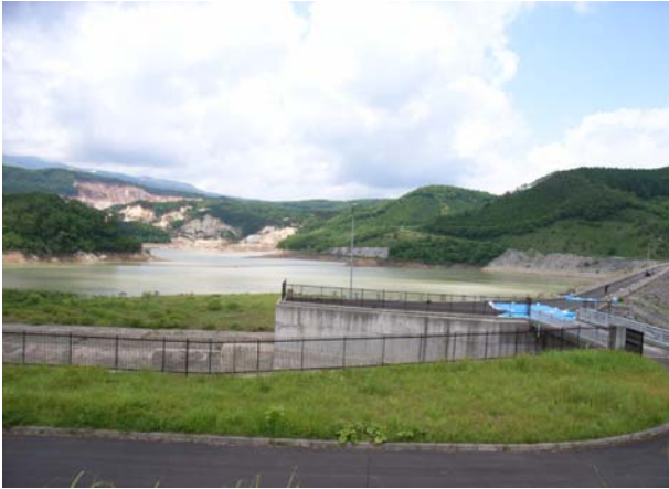
Figure 4. The Aratozawa dam (right) and extensive landslides that occurred upstream of the dam (left)
