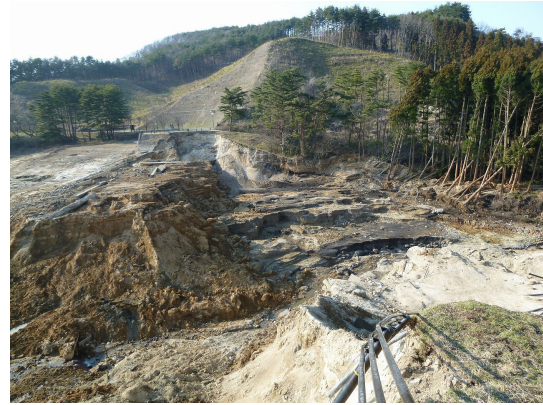
Figure 17. View of breached Fujinuma-ike from right bank
