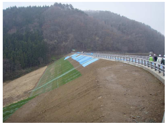
Figure 13. Downstream View of Koromokawa No.1 Dam
