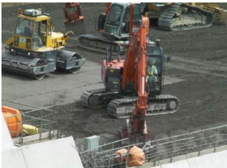
Figure 11. Operational Situation of Slope Edge Compaction
