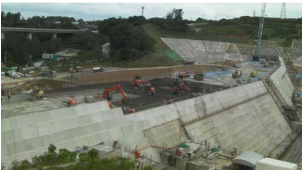
Figure 4. Construction Condition of the Okukubi Dam
