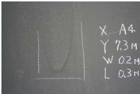
Figure 8. Slope flow in the protection layer
