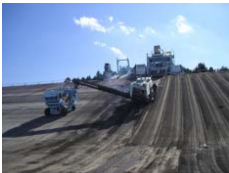
Figure 5. Cutting & removing process
