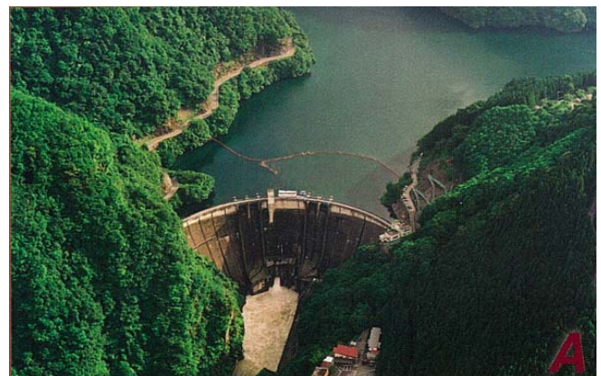
Fig.1. Panoramic view of the Futase Dam
