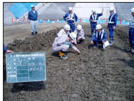
Figure 15. After removing prevention layer (the new method)
