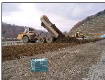
Figure 6. Paving prevention layer (the new method)
