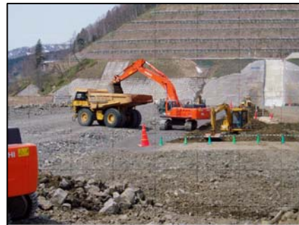
Figure 14. Removing prevention layer (the new method)
