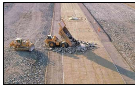
Figure 7. Paving prevention layer (the usual method)
