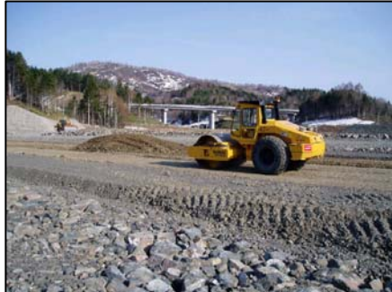
Figure 18. Rolling compaction by vibration roller
