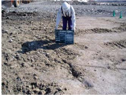
Figure 16. After removing prevention layer (the usual method)
