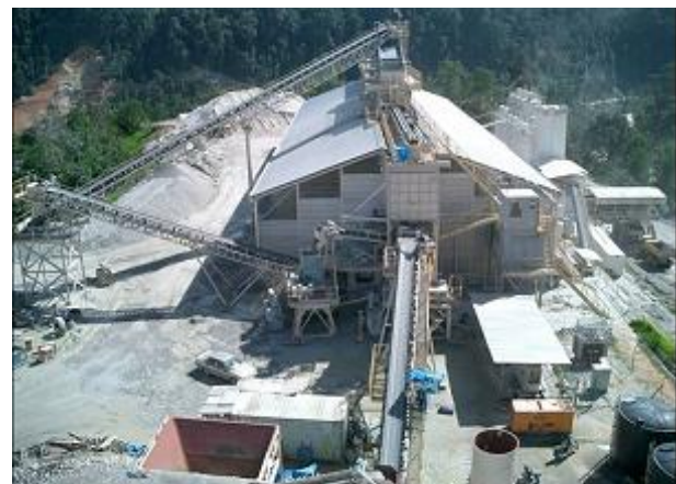
Figure 5. Secondary, tertiary & quaternary crushing plant and products stockpile
