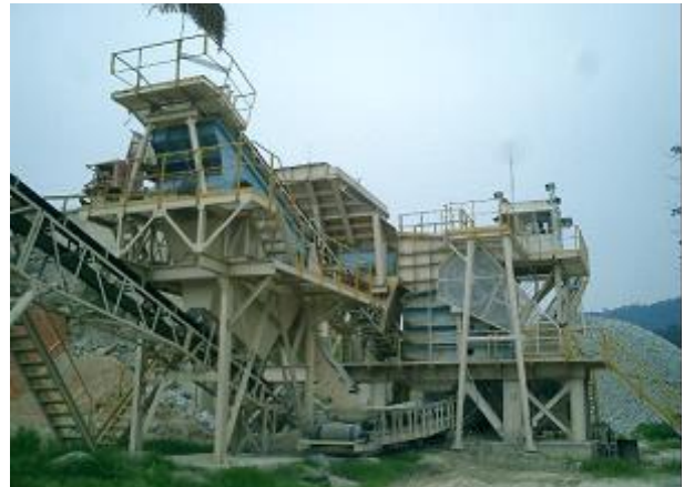
Figure 4. Aggregate plant (Primary crushing plant)
