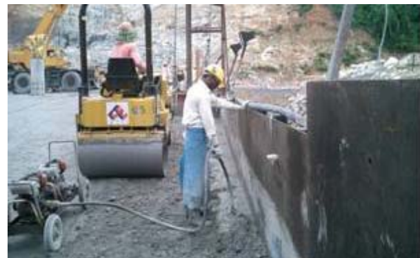
Figure 10. GE-RCC placing
