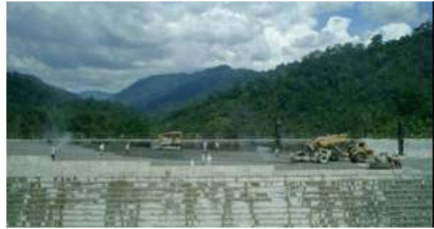
Figure 8. RCC placing by SLM (1)
