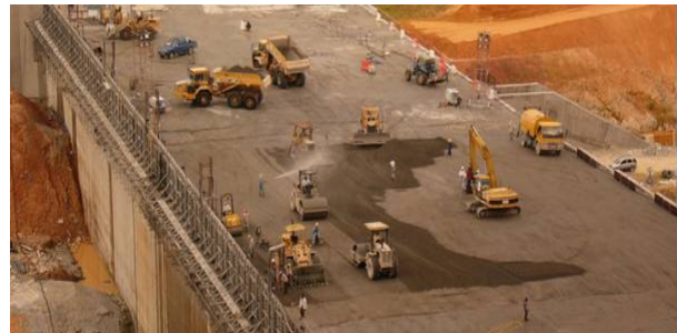
Figure 9. RCC placing by SLM (2)
