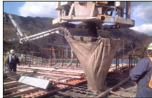
Figure 19. Concreting for the run-off section of the crest road
