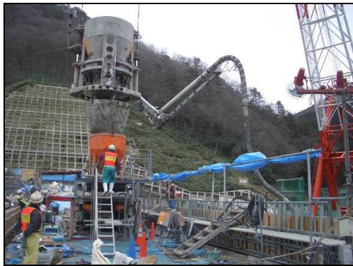
Figure 17. Concrete placement for the overflow section of the dam crest
