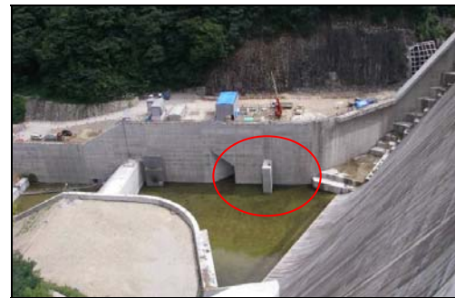
Figure 16. Block to prevent planar eddy currents
