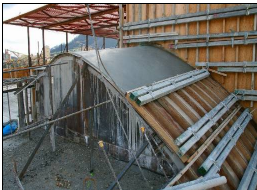
Figure 18. Finishing of the curved overflow section
