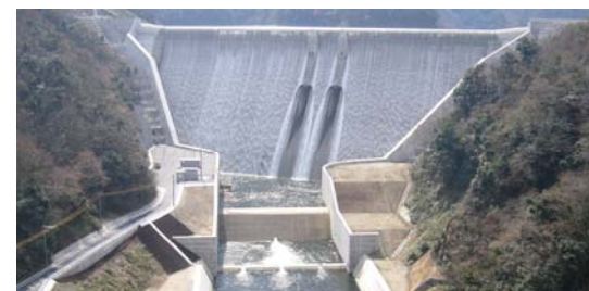
Figure 3. Downstream view of the dam (during overflow)
