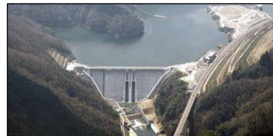
Figure 2. Downstream view of the dam
