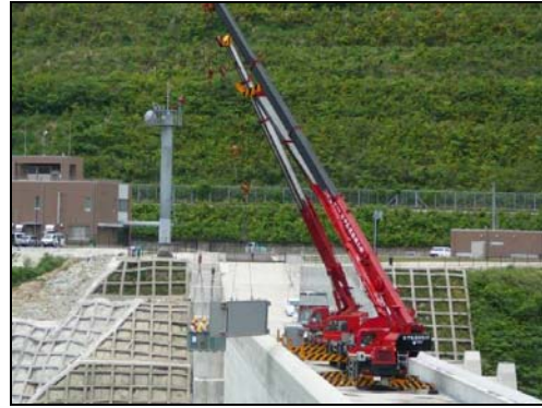
Figure 12. Installation of closure gate for flood control test
