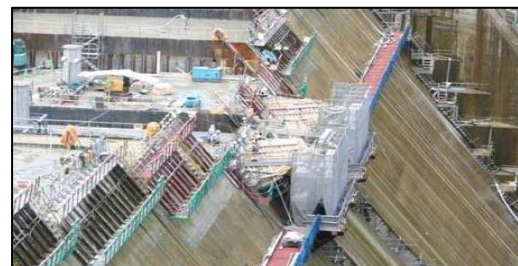
Figure 21. Construction of the deflector above the regulating spillway outlet
