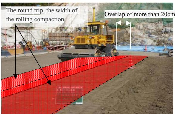
Figure 9. Roller compaction CSG
