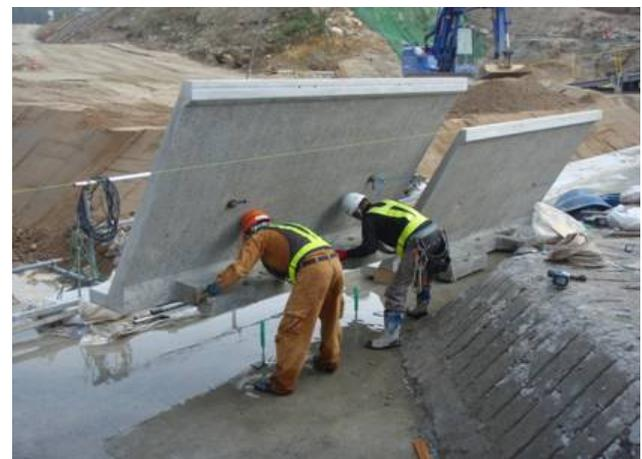
Figure 14. Installation situation of a precast forms
