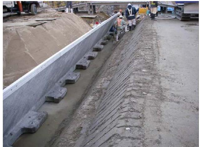
Figure 13. The arrangement situation of precast forms
