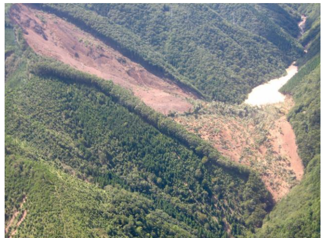
Figure 6. A photo of the landslide dam formed in Nagatono (Taken on Sept. 5, 2011)
