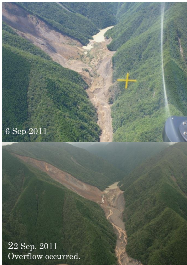
Figure 13. Photos of the Akadani landslide dam Before over flow (above) and after overflow (below)
