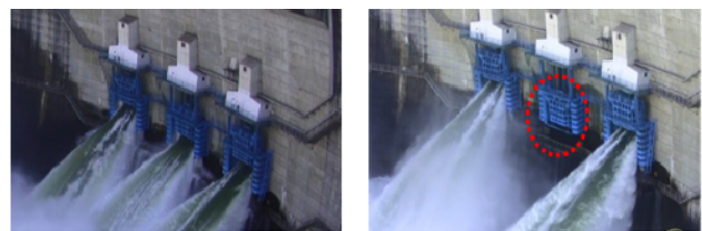
Pattern A (Discharging water from 3 sluice gates)
