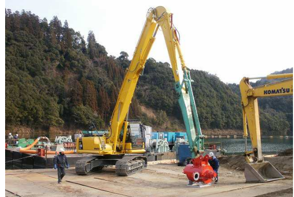
Figure 5. Screw Crusher with Long Arm Excavator
