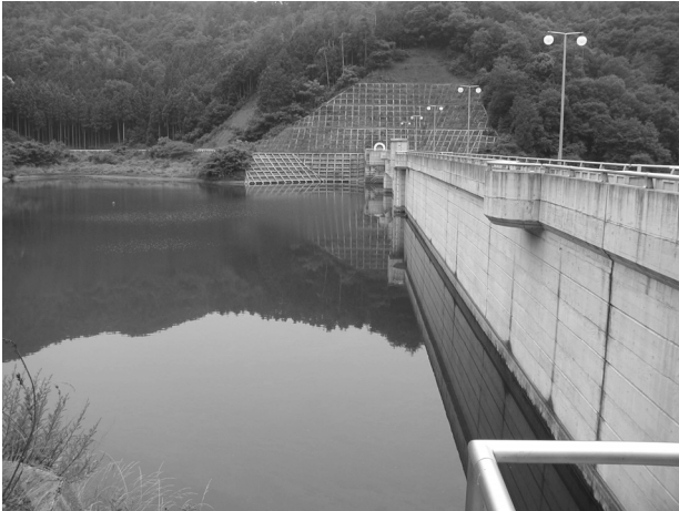
Figure 1. Mitakara dam reservoir.
