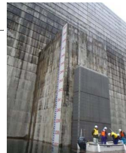
Figure 4. Intake tower of Shitsumi Dam.
