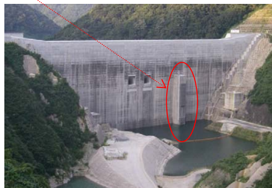
Figure 6. View from upstream and intake tower.
