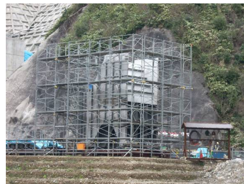
Figure 15. Assembly of an intake tube unit in the assembly yard.
