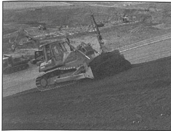
Photograph 4. Levelling by a bulldozer Withures a 3D-MC system.
