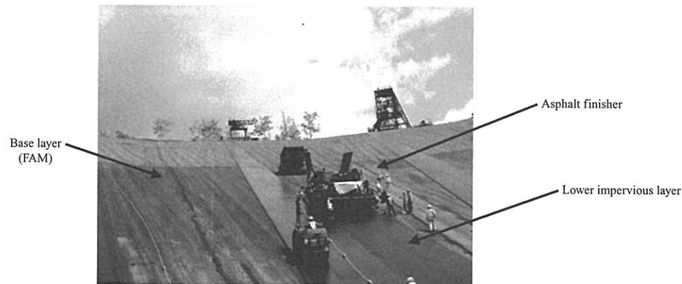
Photograph 5. Situation of the impervious layer.
