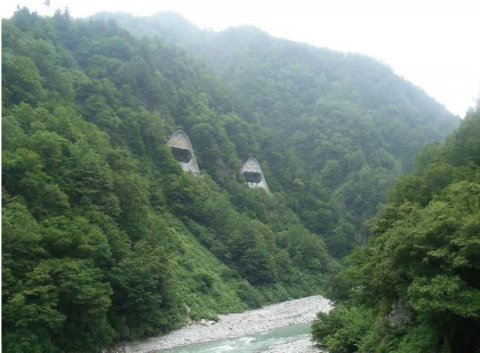
Figure 3. Power line exits of the Kurobegawa No.4 Power Plant.
