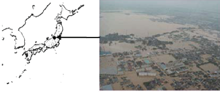
Photo. View of flooding triggered by the breaching of the levee on the Ikarashi river (Sanjo city in Niigata prefecture) (Ministry of land, infrastructure, transport and tourism white paper 2006).
